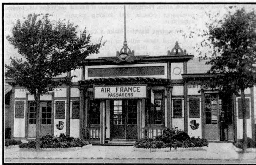
The offices of Air France at Le Bourget. The illustrations are reproduced by courtesy of Compagnie Air-France.
