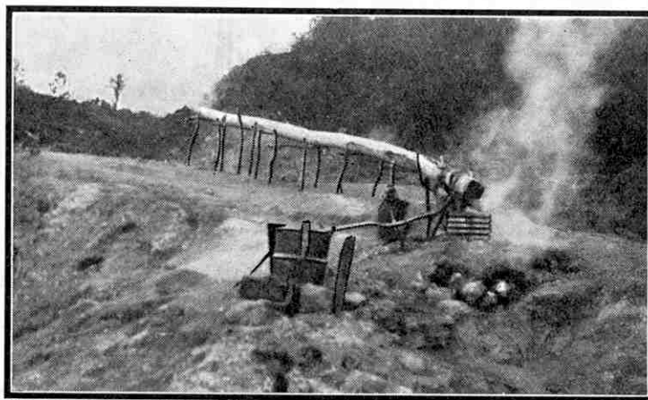
The natural steam collected in the manner illustrated above is passed through long pipes in order to condense it. The water of this unique supply is always warm.
