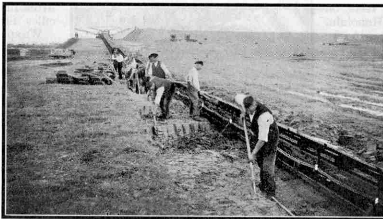
Another view of the plate band conveyor shown above. It runs alongside the surface workings and the workmen dig the coal and load it directly on to the travelling band.
