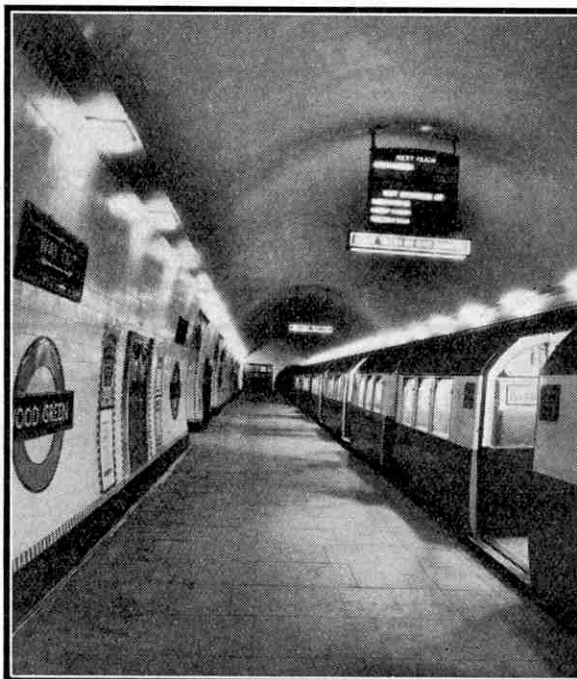
A train at Wood Green Station, on the Piccadilly line. This photograph shows typical "tube" station construction and equipment.
