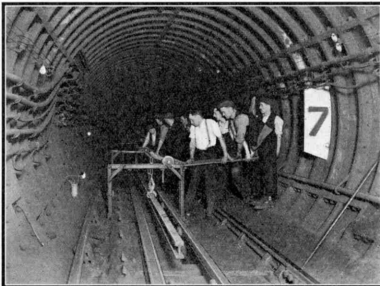
Night work in progress in a London tube, where a rail is being changed. Operations of this kind can only be carried out between the end of one day's service and the beginning of the next.
