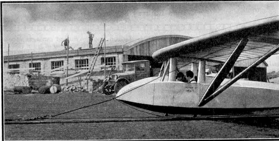
A "Falcon III" two-seater glider about to be launched at Sutton Bank, Yorks. The glider is hauled swiftly along a grooved runway by means of a wire rope attached at one end to the fuselage and at the other to a drum fixed to the back wheel of a jacked-up motor car. The glider rises rapidly, and when it is sufficiently high the rope is released. Photograph by J. H. Illingworth, Harrogate.
