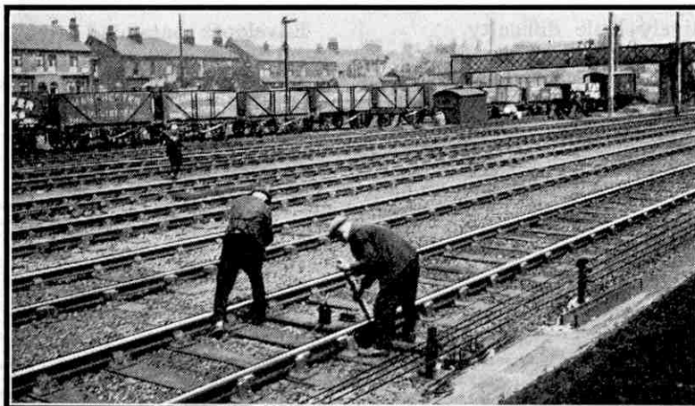
Helping to maintain the permanent way in first-class order near Patricroft. The platelayers are removing fishplates to be oiled so that the rails can slide along them easily when expanding or contracting. (H.R.C. prize-winning photograph by F. Hodson, Bolton.)
