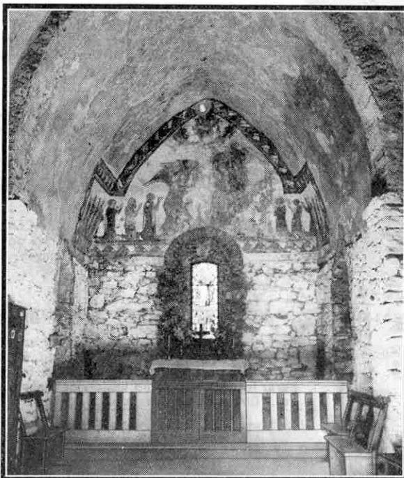
The Fisherman's Chapel, La Corbière, Jersey. The interior is painted with pigments made from seaweed and the colours show clearly only in rainy weather. Photograph by G. P. Warner.
