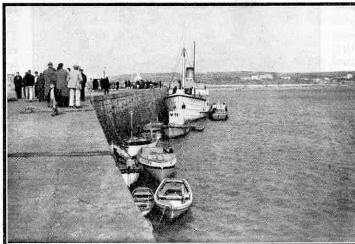
The Hugh Town pier, St. Mary's. This is built out into St. Mary's Pool, and stretches from the shore to a rocky islet in the bay.
