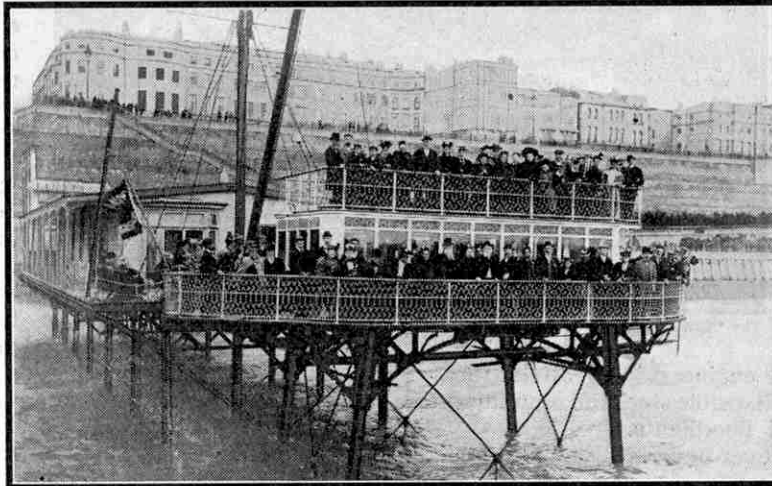
An electric railway, designed and built by Magnus Volk, which for a time ran through the sea at Brighton. The illustrations to this article are reproduced by courtesy of Magnus Volk Ltd.
