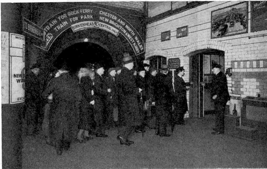
Passengers entering one of the new lifts of the Mersey Railway, the largest high speed lifts in Great Britain. The illustrations to this article are reproduced by courtesy of Wm. Wadsworth and Sons Ltd., Bolton.
