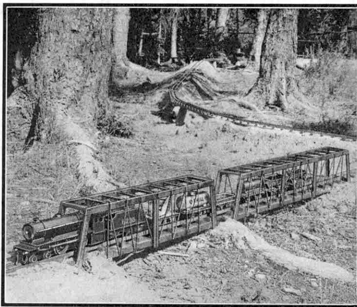
An interesting view showing the miniature line passing through thickly wooded country. This illustration shows how the protruding roots of trees that would cause an obstruction are avoided by means of specially constructed steel truss viaducts.
