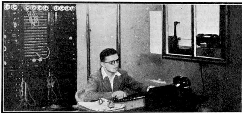
The mixer at work in the dubbing theatre, where the final sound track on a film is built up from its components.
