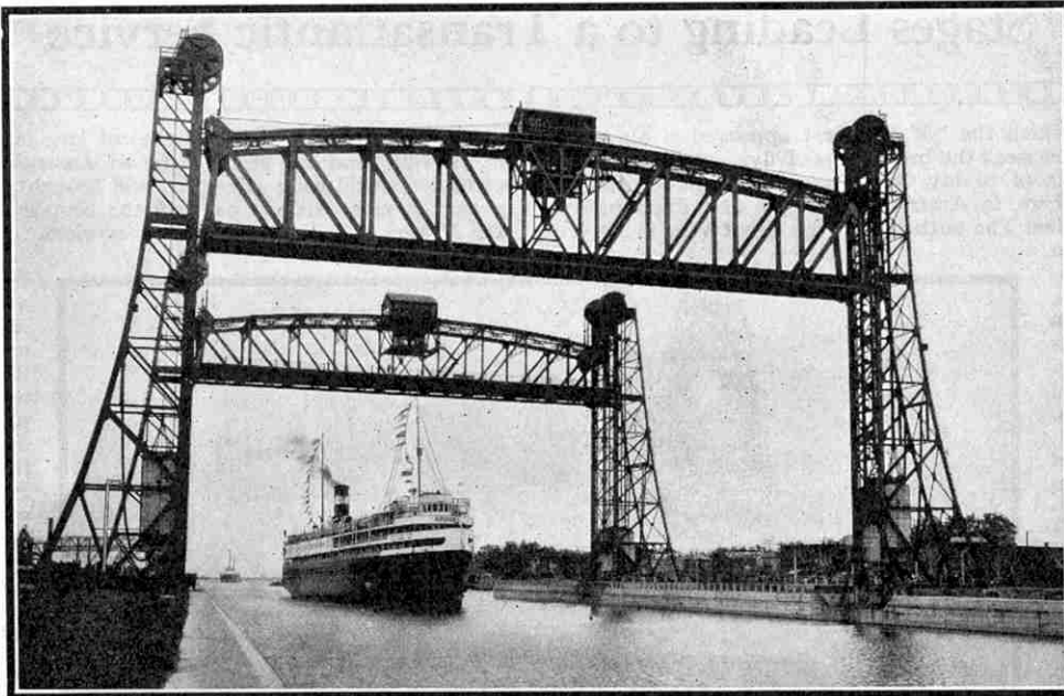
Two of the eleven vertical lift bridges that cross the Welland Canal, with their spans shown in the raised position.
