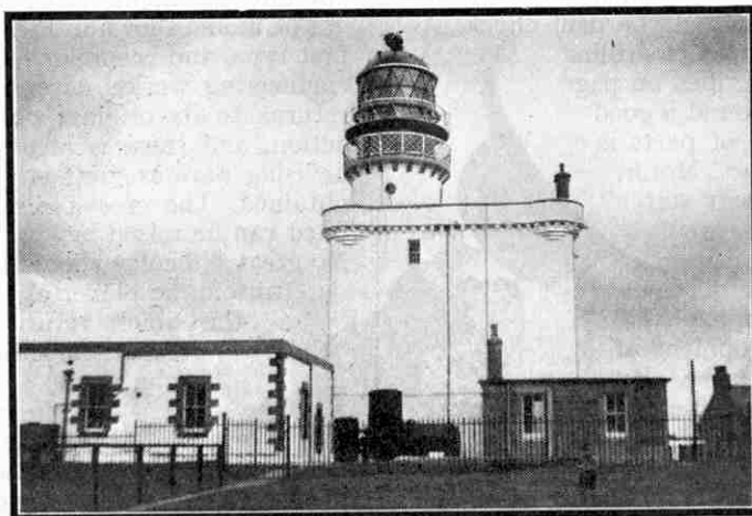
Kinnaird Head Lighthouse, Aberdeenshire. The tower is that of an old castle. Photograph by Rev. R. I. Mitchell, Lonmay.
