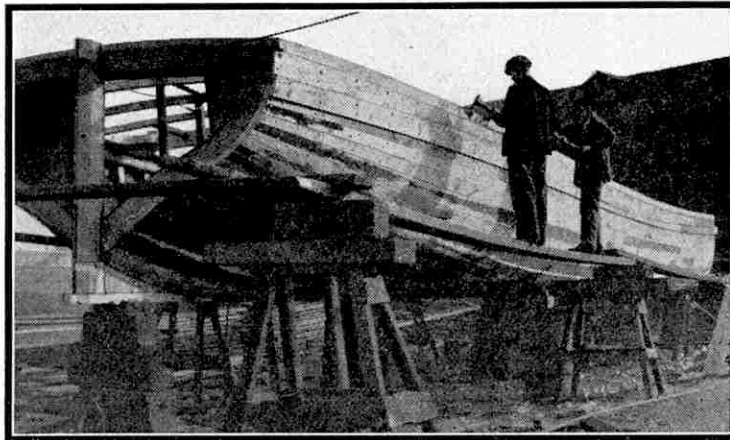
Carpenters engaged in adze work on a barge on the stocks.
