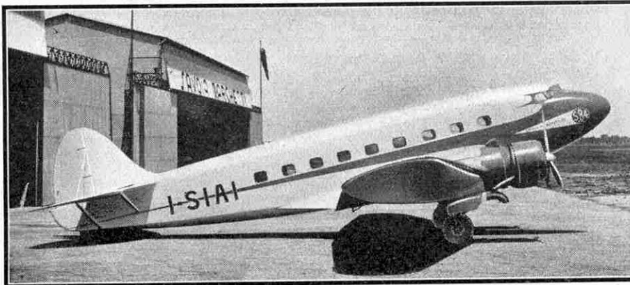
The Savoia-Marchetti S-84, a twin-engine monoplane air liner with seating for 18 passengers.
