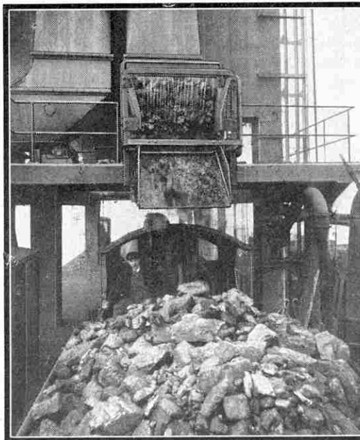
The modern method of coaling. The fuel being fed to the tender from an overhead bunker. Photograph by courtesy of the L.M.S.
