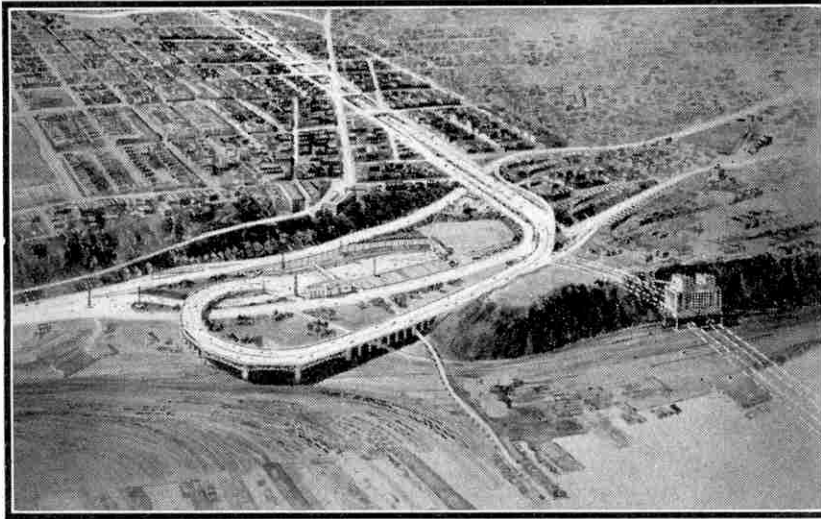
The ultimate arrangement of the New Jersey approach of the Lincoln Tunnel, showing the loop viaduct and the depressed road now being constructed. One of the ventilation buildings also can be seen.
