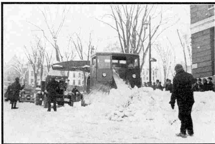
The Joy Snow Loader at work removing a large heap of snow and ice, which it is loading into a lorry standing alongside.
