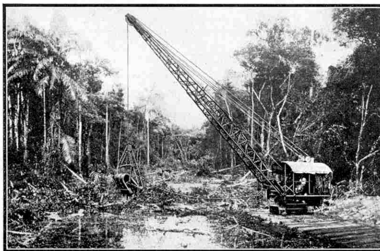
Typical working conditions in the swampy Malayan jungle. The weight of the excavator is supported by a mattress of timber that is moved along with it by chains attached to the scoop.
