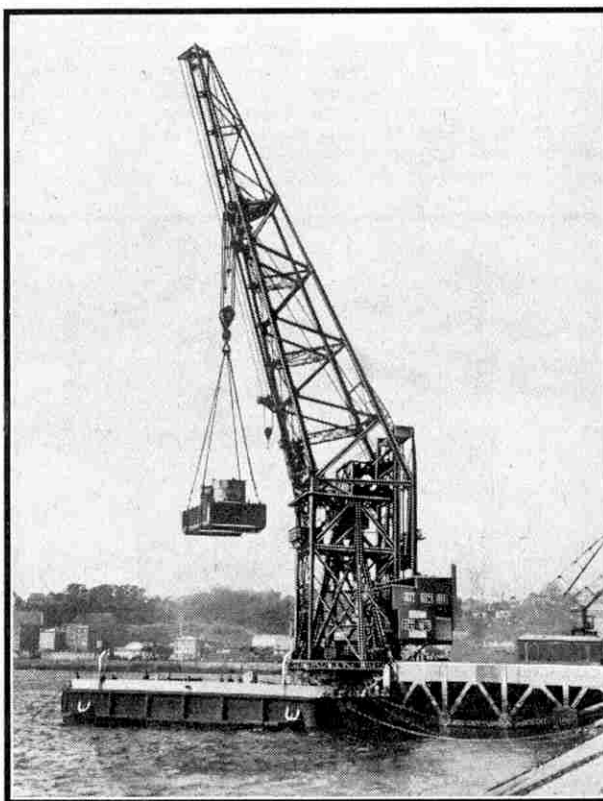
The world's largest Diesel-electric floating crane lifting 250 tons in Brest Harbour. Photograph by courtesy of Demag A.G., Duisburg, Germany.
