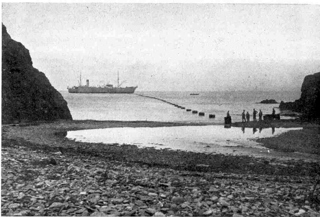
Landing the shore end of the Wales-Eire cable at Nevin from the cable ship "Faraday." The cable was floated ashore on barrels. For the illustrations to this article we are indebted to Siemens Brothers and Co. Ltd., Woolwich.
