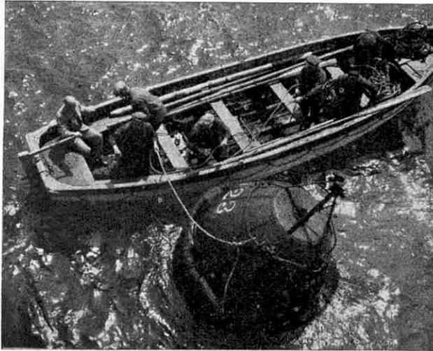
Recovering a mark buoy during the laying of the Anglo-Dutch cables.
