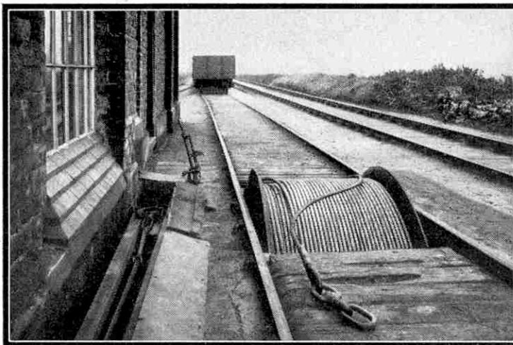
The winding drum at the top of the incline at Swannington. This photograph shows the coupling by means of which the wagons are attached to the cable.
