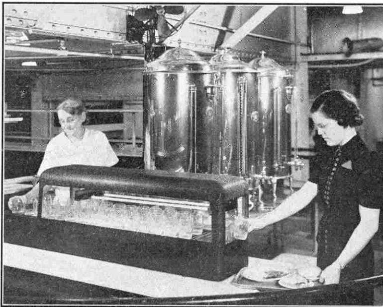
Sterilizing drinking glasses by means of Sterilamps. The ultra-violet rays from the long tubes destroy bacteria on the glasses in the installation. Photograph by courtesy of the Westinghouse Electric and Manufacturing Company, Pittsburgh, U.S.A.
