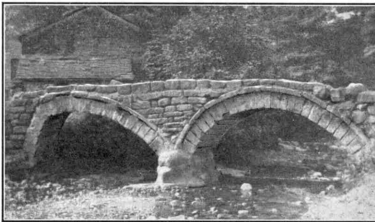
The pack-horse bridge at Wycollar, near Colne, Lancashire. Bridges of this kind are narrow, with low parapets to allow room for the bulging panniers of the pack-horses.
