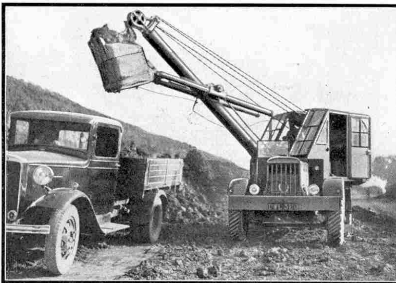
The Allen mobile mechanical excavator described on this page loading material into a lorry for removal. Photograph by courtesy of John Allen and Sons (Oxford) Ltd., Cowley, Oxford.
