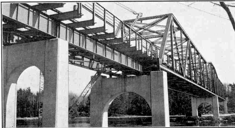
The continuous truss span that crosses the channel between Hill and Constance Islands, two of the stepping stones in the St. Lawrence used by the builders of the Thousand Islands Bridge. The central pier rests on a rock island in midstream.
