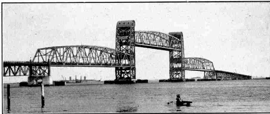
The three central spans of the bridge, each with a length of 540 ft. The central span weighs 2,180 tons and electric motors raise it 95 ft. in two minutes.
