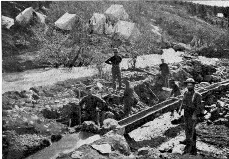
Sluicing in progress in the Alaskan goldfields. The man with the spade is Gold Nugget Charlie, the story of whose life is reviewed on this page.
