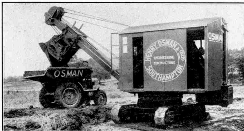
A Smith multi-purpose excavator equipped as a skimmer scoop for removing top soil. The machine can easily be converted for work as a grab crane, trench digger, navy or dragline. The illustrations to this article are reproduced by courtesy of Thomas Smith and Sons (Rodley) Ltd., Leeds.
