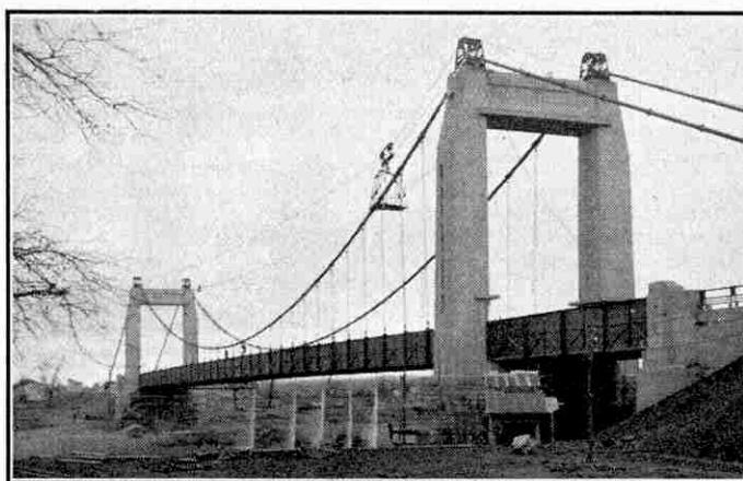
Water pouring from the flooded roadway of the Aiguilly bridge after the novel water test described on this page had been completed. The photographs on this page are reproduced by courtesy of M. Lambert, Roanne (Loire), France.
