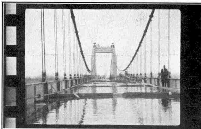
A photograph of the flooded roadway of the Aiguilly bridge taken during the tests. The water fills the tanks built on the bridge.
