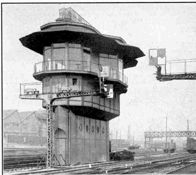
A steel signal cabin at St. Denis, near Paris, with lattice structures bringing signals directly over their tracks. This illustration and the lower one on the next page are reproduced by courtesy of "The Railway Gazette."
