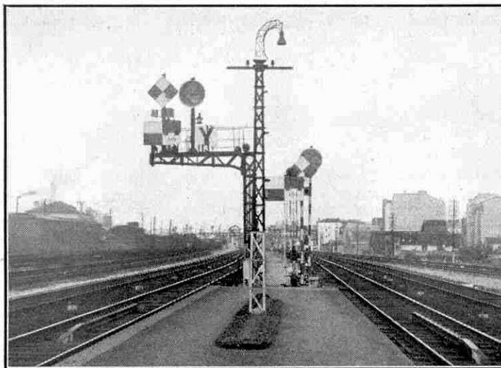
A selection of French signals on the State Railways. These include the carré , or red and white chessboard, and the red disc mentioned in this article. The ramps in the tracks are for cab signalling purposes. Photograph by courtesy of Mr. T. S. Lascelles.
