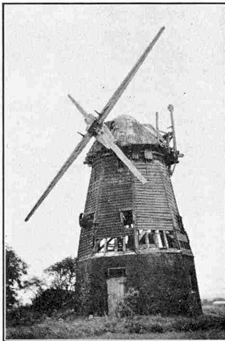
A smock mill in decay. This photograph shows the mill at Stapleford, Cambridgeshire.
