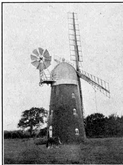
Barnham mill, Suffolk, a tower mill with a fantail to bring the main sweeps into the wind. Sails and fantail are carried by a revolving head.
