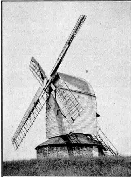
Drinkstone mill in Suffolk. This probably is Britain's oldest working windmill, and is a good example of a post mill with a roundhouse.
