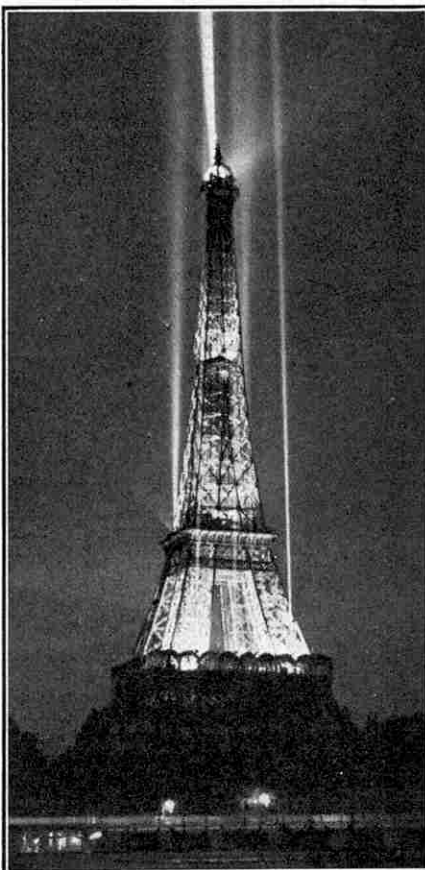
The Eiffel Tower illuminated for the International Exhibition in Paris in 1937, when it could be seen at night from a distance of more than 60 miles. Photograph by courtesy of "Le Dimanche Illustré," Paris.
