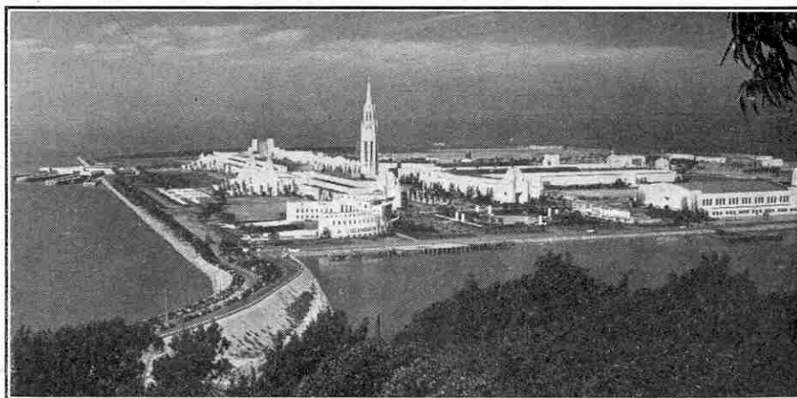
The unique island on which the San Francisco International Exposition is being held. It was built up by pumping black sand from San Francisco Bay into a space enclosed by a sea wall three miles long. The Tower of the Sun in the centre of the exhibition is 400 ft. high and a carillon with 44 bells is mounted on it.
