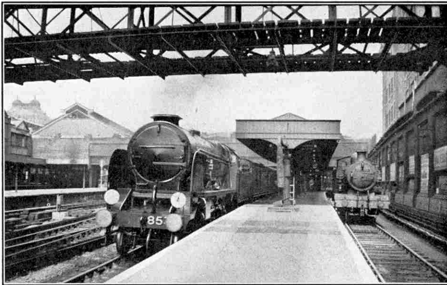
S.R. locomotive "Sir Richard Grenville," showing the large diameter of the chimney that is required by the Lemaître multiple-jet blast pipe arrangement fitted to this and several other S.R. locomotives.
