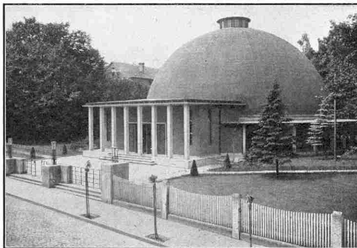
Outside the Jena planetarium, which was the first to be built.
