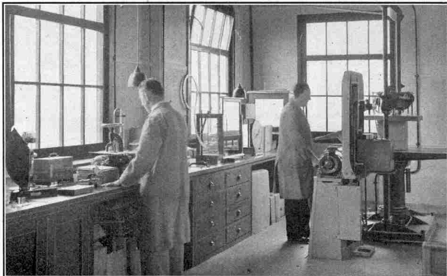
Another corner of the laboratory. On the right is a machine that tests the resistance of boxes to weights placed on them.
