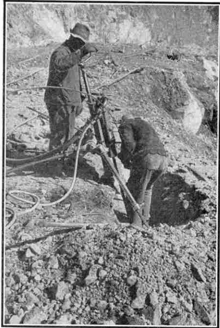
Drilling deep holes for blasting in an asbestos mine.
