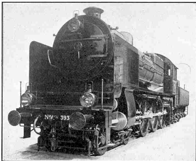
The heaviest engine in service on the railways of Holland.
