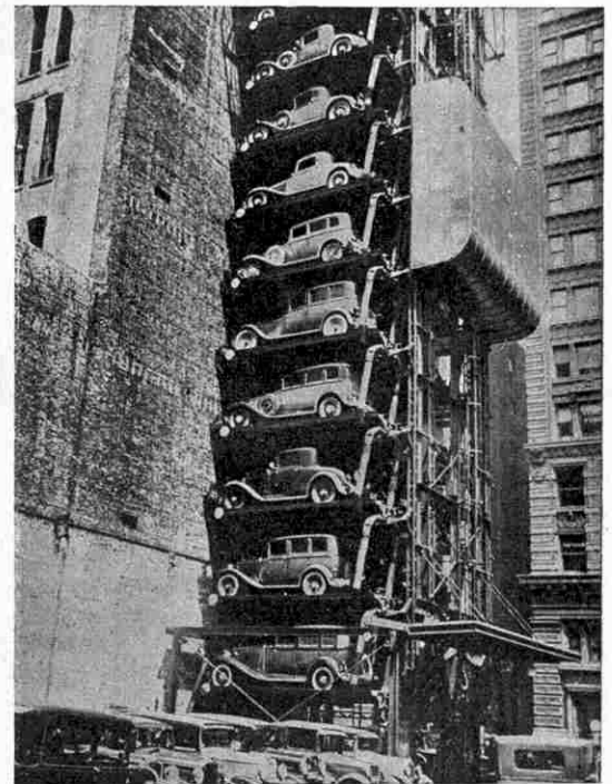
A motor car parking place built like a skyscraper. From "The Highway," reviewed on this page.
