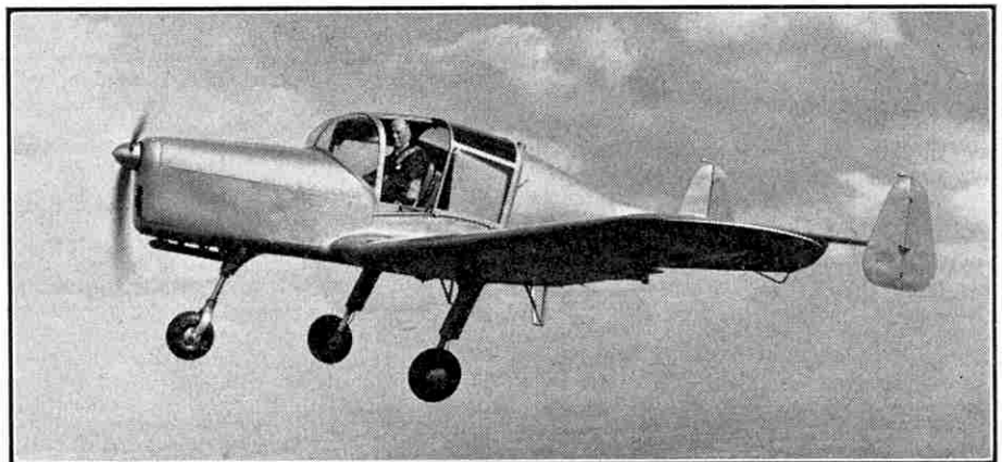
The G.A. "Cygnet," a British two-seater all-metal monoplane fitted with a tricycle type undercarriage. Photograph by courtesy of General Aircraft Ltd.
