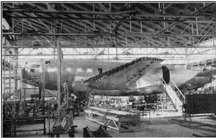
The Curtiss-Wright Sub-stratosphere monoplane under construction in the St. Louis factory of the Curtiss-Wright Corporation. It is designed to carry 30 passengers and 6,000 lb. of mail and freight, and is the largest twin-engined air liner ever produced in the United States of America.
