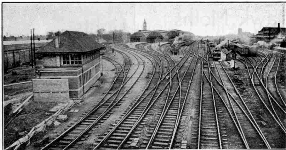
Darlington South End, showing new signal box on left and main lines passing straight outside the station.
