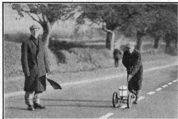
The "Invicta" road line marker. Photograph by courtesy of Aveling-Barford Ltd., Grantham.
