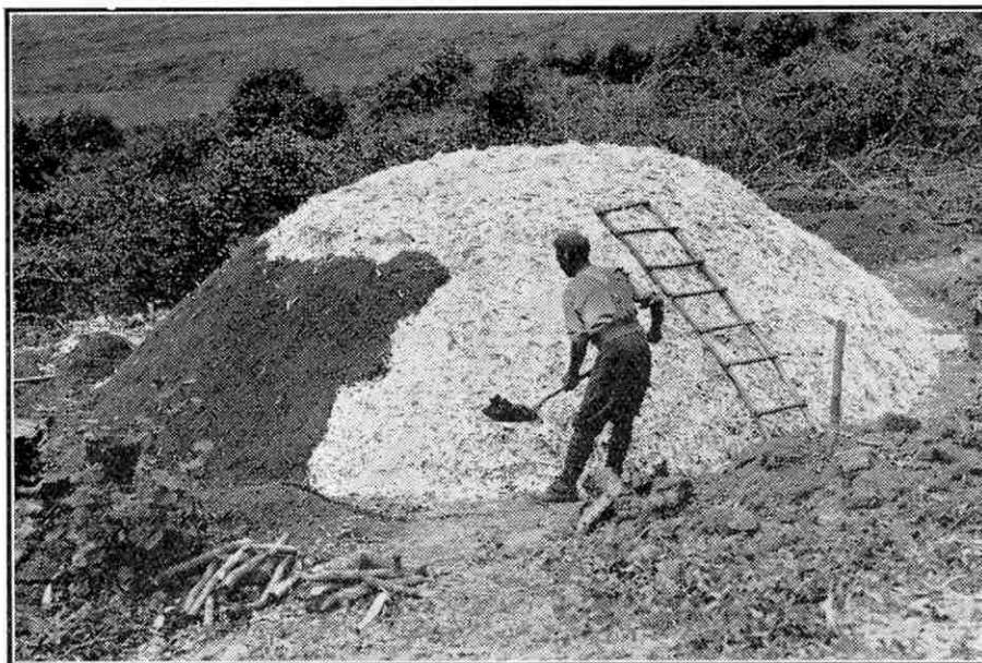
A charcoal burner covering his pile of logs with earth before setting the mass alight.
