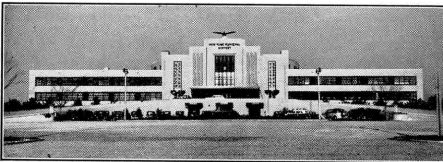
The imposing front of the landplane administration building, showing the motor traffic circle and ramp that provide for discharging and loading passengers at two levels of the terminal.
