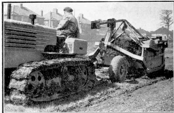
Fig. 3. Scraper with full load ready to be hauled to the discharge point.
