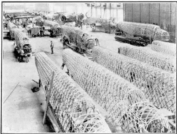
Geodetic fuselages of Vickers "Wellington" bombers. Photograph "The Aeroplane" Copyright.
