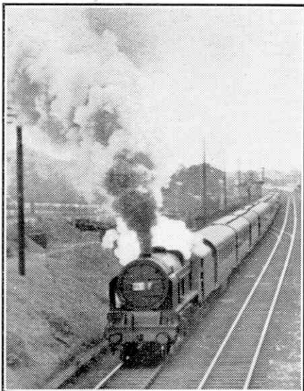
When one track is under repair trains have to proceed, under special rules, on the wrong road. Our photograph shows an L.M.S. Scottish express in these circumstances. Photograph by W. S. Garth, Luton.
