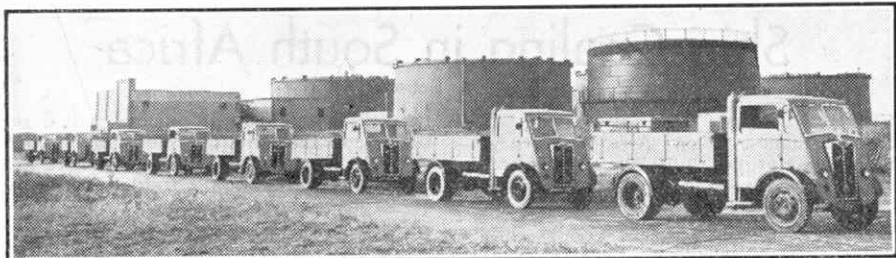
Guy "Vixen" lorries of the Croydon Borough Council that run on methane produced from sewage.
