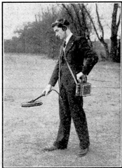
Tracing underground pipes with the "Cintel" Metal Detector. Photograph by courtesy of Cinema Television Ltd.
