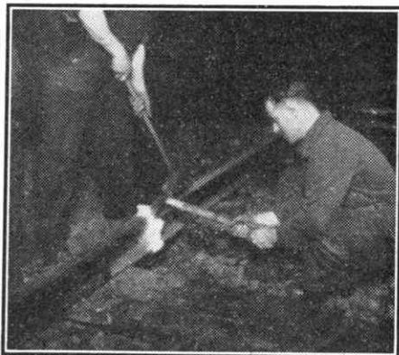
Trimming off excess of thermit steel.
