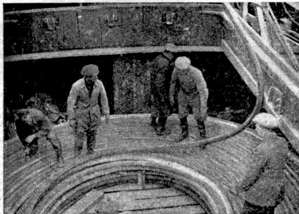
Cable laying from coil.
