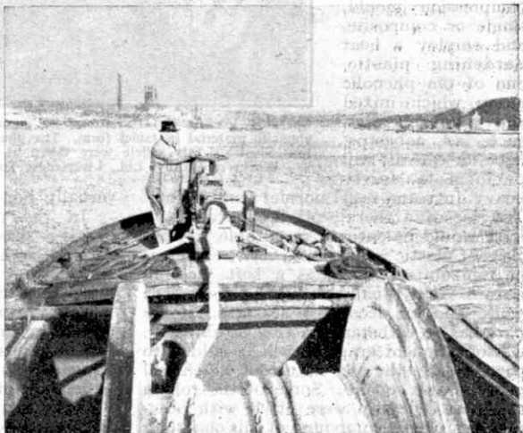
Cattewater: Cable laying from drum.
