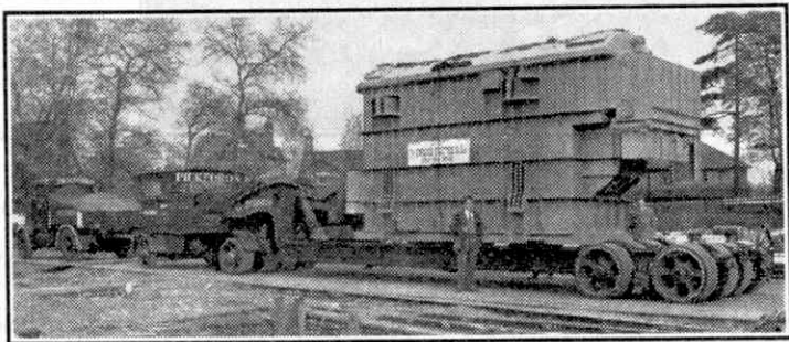
A 45,000 kVA 132/33 kV transformer for the Central Electricity Board, leaving Stafford by road for Nottingham. Photograph by courtesy of the English Electric Company Ltd.
