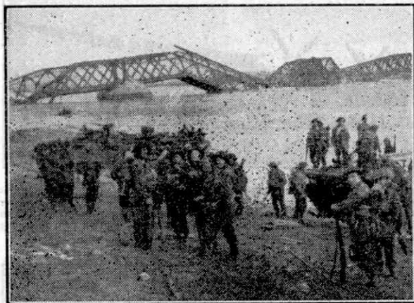
A scene on the banks of the River Rhine near a demolished railway bridge. Every bridge over the Rhine in the British Zone of Germany was destroyed. British Official Photograph, Crown Copyright Reserved.
