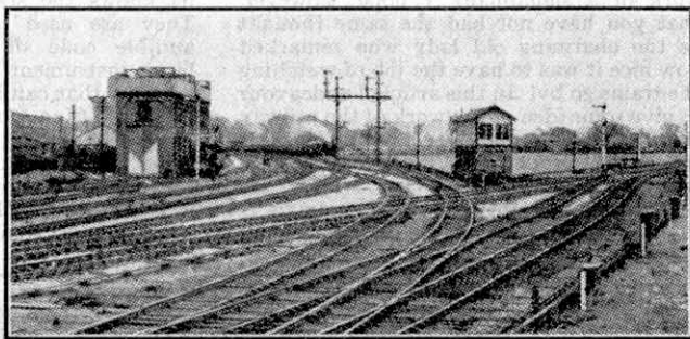
An important main line junction and the signal box controlling it. The signalman here is well placed to observe traffic movements on each route. Photograph by courtesy of the L.M.S.
