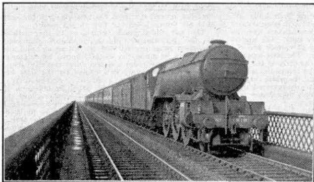
Crossing the Tay Bridge, on the L.N.E.R., the longest in Britain. The train is an Aberdeen express hauled by "V2" 2-6-2 No. 819. Photograph by H. C. Casserley.
