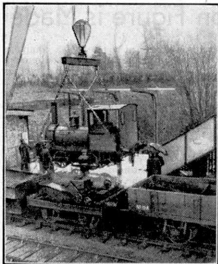
The veteran "Shannon" of the Wantage Tramway being lifted into position for preservation at Wantage Road station, Western Region. Photograph by H. J. Milligan, Abingdon.
