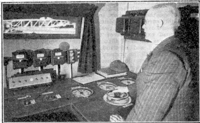
The control room for the working of the road machine.
