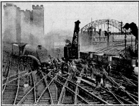
An up express from Edinburgh picks its way along the only track left open during the renewal of the crossings near the High Level Bridge at Newcastle. British Railways Official Photograph.
