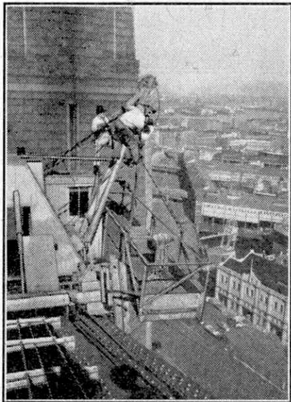
Sidney Black and Ernest Tomrup are quite at ease overhauling the hoisting wires of a painting stage 250 ft. above sea level.
