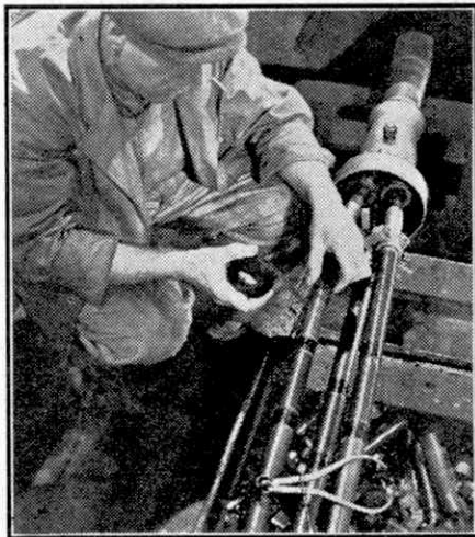
A cable jointer at work on a straight connection.
