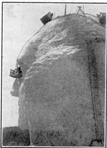
This side view of the Washington head shows how deeply the rock had to be cut away to prepare for the next figure, and how the work was carried out.
