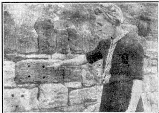
Stone sleepers that probably were used on the former Storeton Tramway. Photograph by C. R. Rowson, Liverpool.
