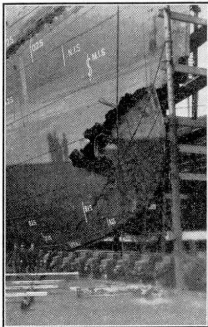
The bow of the American liner "St. Paul" torn by her collision with H.M.S. "Gladiator."
