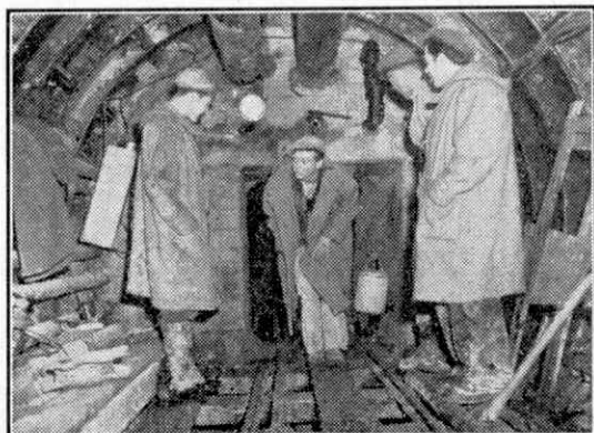
Miners coming out of the entrance air lock after finishing an 8-hr. shift in the pressurised tunnel.
