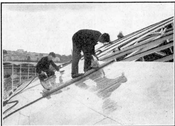
Laying aluminium sheeting on the roof of the Dome of Discovery.
