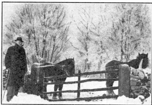
How a gateway is fitted into a drystone wall.
