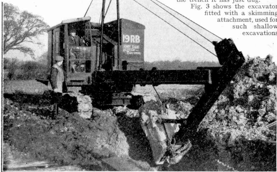
Fig. 1. Mechanical excavator working as a "back acter."
