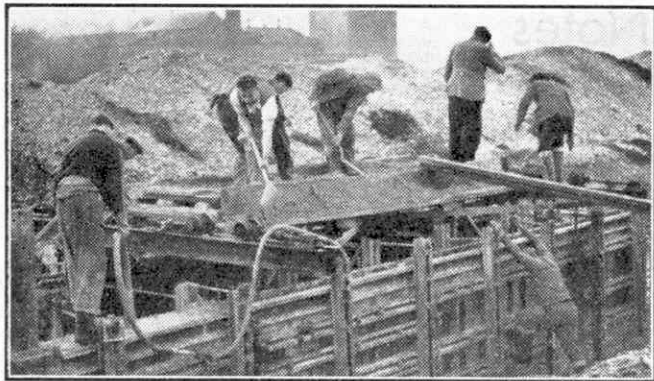
Fig. 8. Reinforced concrete storm water culvert under construction.
