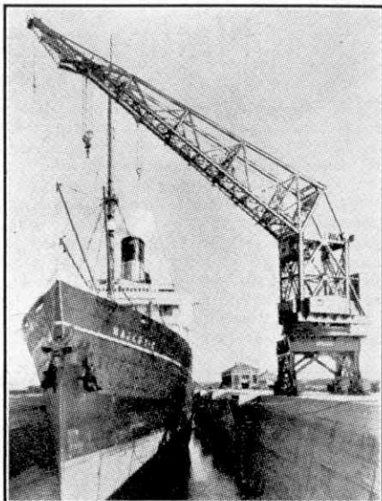
An electrically-operated screw luffing crane installed at Southampton for dry-dock service. Its maximum load is 50 tons.
