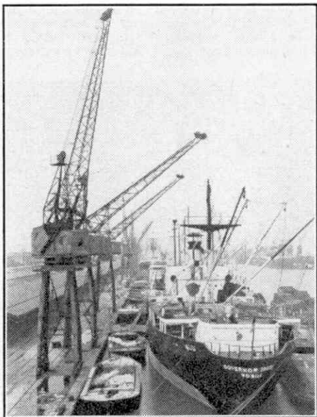
Dockside cranes at work. For the illustrations to this article and for the photograph on which our cover is based we are indebted to Stothert and Pitt Ltd., Bath.
