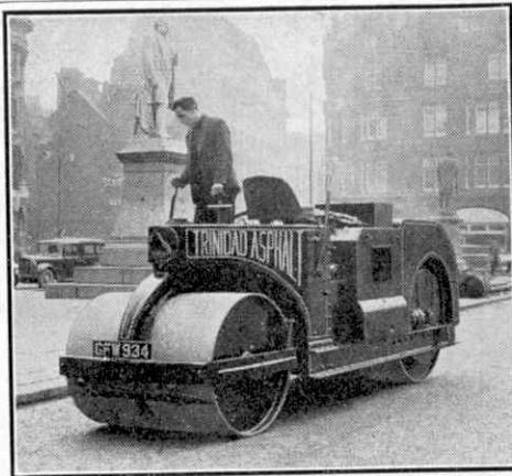
A modern tandem diesel road roller at work in Albert Square, Manchester. The driver is looking backward. It is a product of Marshall Sons and Co. Ltd., Gainsborough, to whom we are indebted for our photograph.
