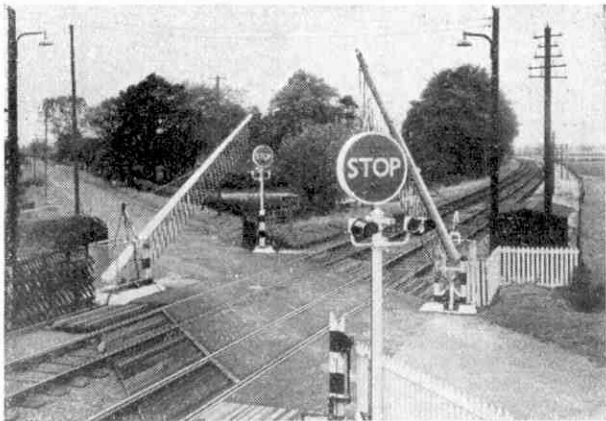
A level crossing barrier that reminds us of those to be seen in the United States and Canada. It is an experimental lifting barrier, with "Stop" lights and boards and floodlighting, that has been installed at Warthill, Yorkshire, on the N.E.R. line between York and Hull.
