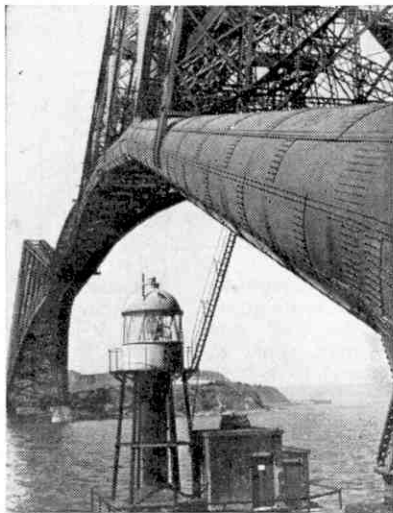
The central cantilever of the Forth Bridge rests on the island of Inchgarvie, on which the lighthouse seen in this picture has been erected as a guide to shipping. British Railways Photograph.
