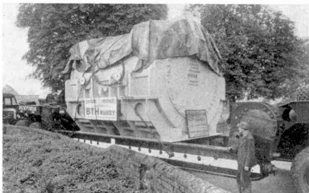
Stator of the BTH 25,000 kW hydrogen-cooled turbo-alternator for Canada, en route from the BTH Works at Rugby to Liverpool Docks. The weight of the load was 109 tons. Photograph by courtesy of British Thomson-Houston Co. Ltd., Rugby.
