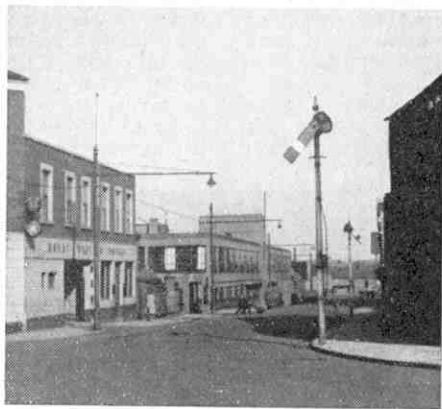
A railway signal by the roadside. It protects a level crossing in Worcester. Photograph by E. H. Sargeant, Birmingham.
