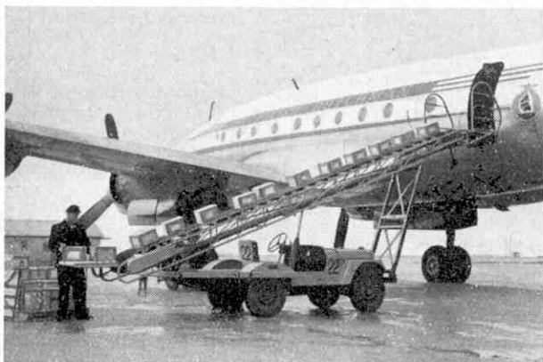
A Jeep converted into a mobile loading ramp in use at K.L.M.'s airport at Schiphol. Photograph by courtesy of K.L.M. Royal Dutch Airlines, London.
