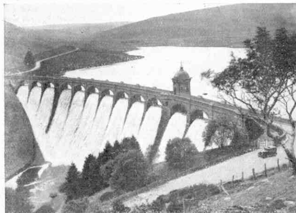
Craig Goch Reservoir, one of the three originally constructed in the Elan Valley, Radnorshire, to supply Birmingham with water. Photograph by courtesy of the City of Birmingham Information Department.
