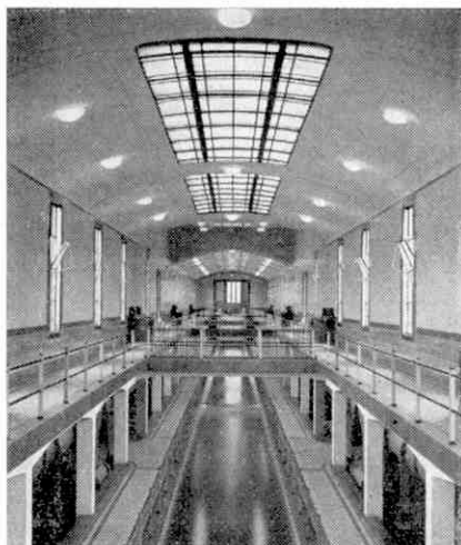
Inside the primary filter house at Hampton Waterworks. Metropolitan Water Board photograph.
